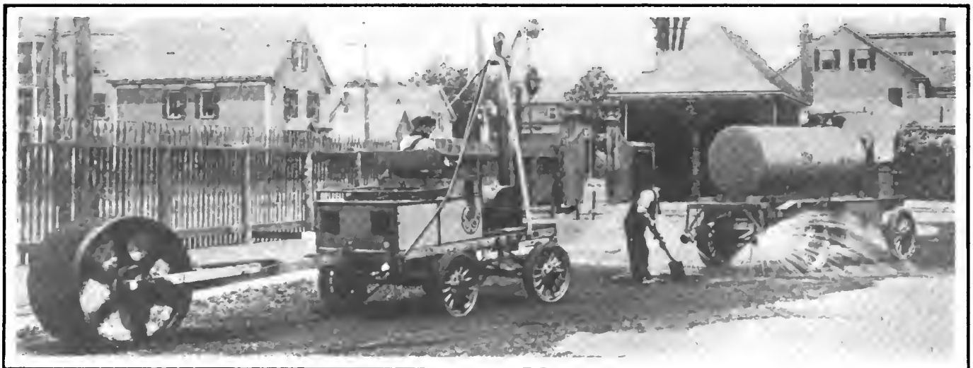
Two applications of the electric to municipal work. At the left is a one-ton machine used in road making and at the right a street sprinkler. The crane on the former may be used for laying curbing or flagging, installing fire hydrants, etc.
